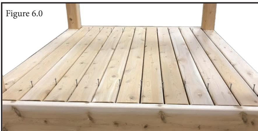
Figure 6.0 Shows how to use the screws for spreading out deck boards with even spacing.
